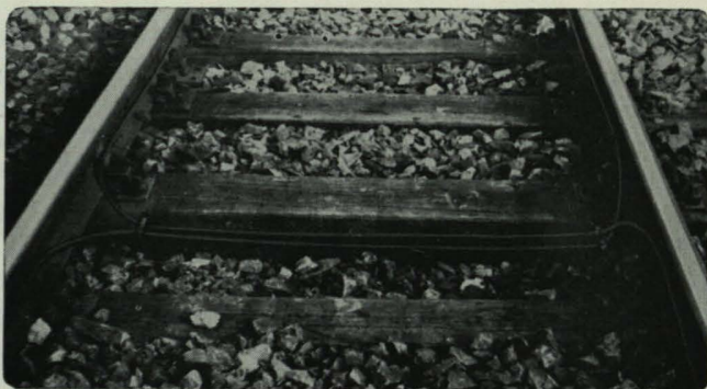
Fig. 6 Cables used for inductive train communication
