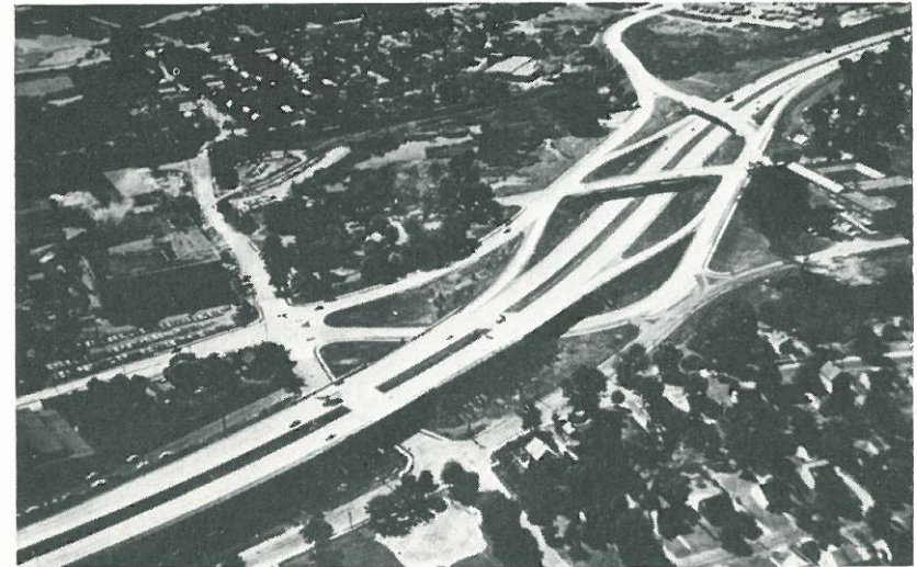
FIG. 1. An interchange on the Connecticut Turnpike (U.S.A.)
