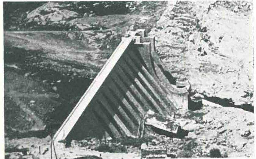
FIG. 12. Vega de Terra Dam, Spain, after failure
