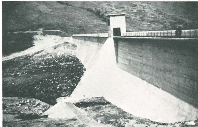
FIG. 10. Allt na Lairige Dam (prestressed dam), Scotland
